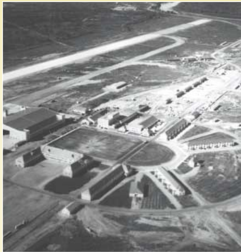
North Post and runway, ca. 1942. Clockwise around parade ground from Hangar One on the left: Service club/bus station, power plant, quartermaster, 2 NCO quarters, commander's house, officers' quarters, garage, BOQ barracks/BX/hospital. Rail facilities, access road and warehousing are visible in upper right.
