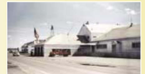
Ladd Field Fire House (and Rescue Unit), north side of Quartermaster building. University of Alaska, Fairbanks, Cecil H. Kornegay Photograph Collection, 1946-1948 UAF-1999-204-112
