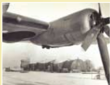
B-24 with engine heater (duct) at 35°F below.
