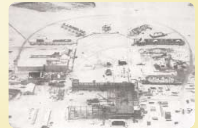
An aerial view of the Headquarters area in 1940. Hangar No. One is under construction in the foreground, while the foundation was being laid for the Air Corps Barracks, and the BOQ was receiving finishing touches. AAF photo.
